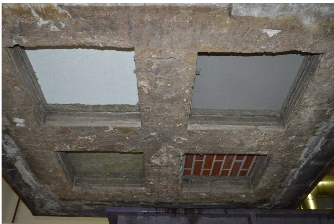
Photo No. 1 Test specimens no 1, 2, 3 and 4 from exposed side before test (test 1)
